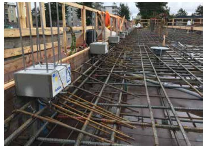
Fig. 4: Thermal breaks for parapets are installed at the vertical wooden parapet forms and tied into the horizontal reinforcing bars. Reinforcing bars are fabricated to transfer both bending and shear across the insulation layer
