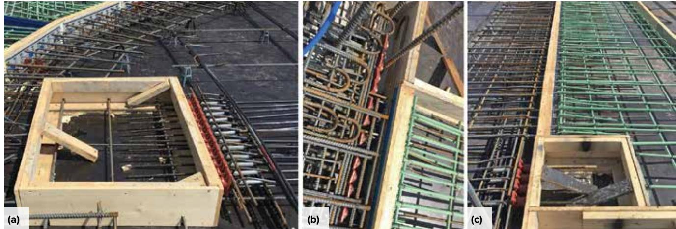
Fig. 5: Structural thermal breaks can be installed in post-tensioned slabs: (a) a blockout within the slab; (b) a thermal break at dead ends of tendons; and (c) a blockout within a balcony. In the latter case, the opening can be filled using rigid insulation and concrete
