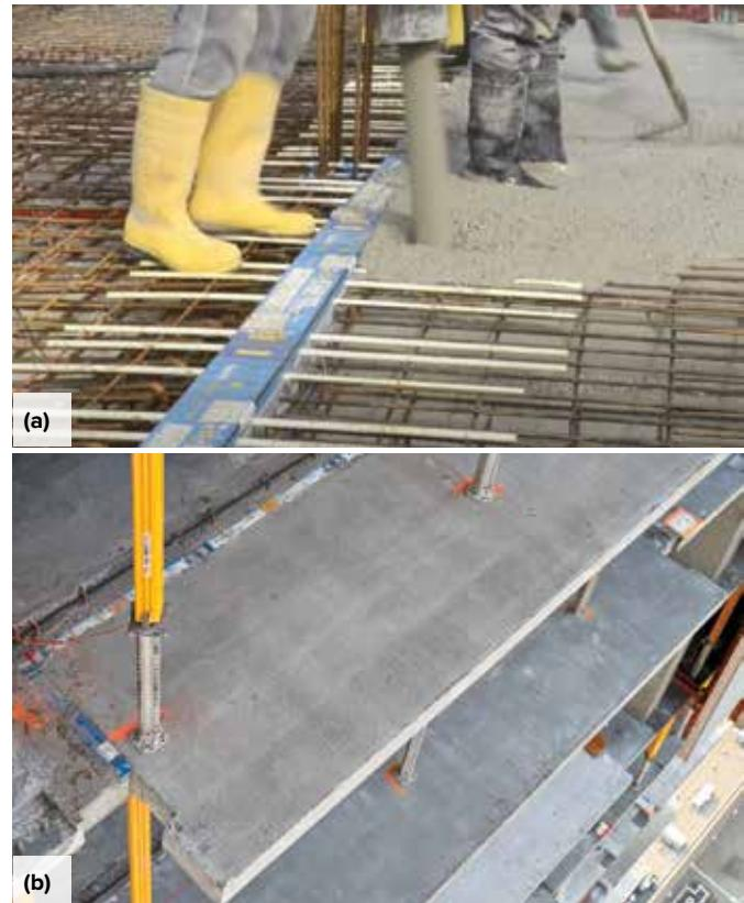
Fig. 3: Structural thermal breaks in balconies: (a) during placement of balcony concrete; and (b) after placement of balcony and slab concrete. Note: Modules are installed with the top plate flush with the exterior concrete structure. The white bars are GFRP bars
