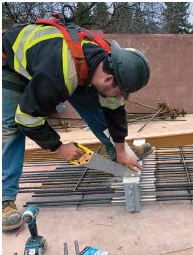
Fig. 2: A thermal break module may be cut with a handsaw if required
