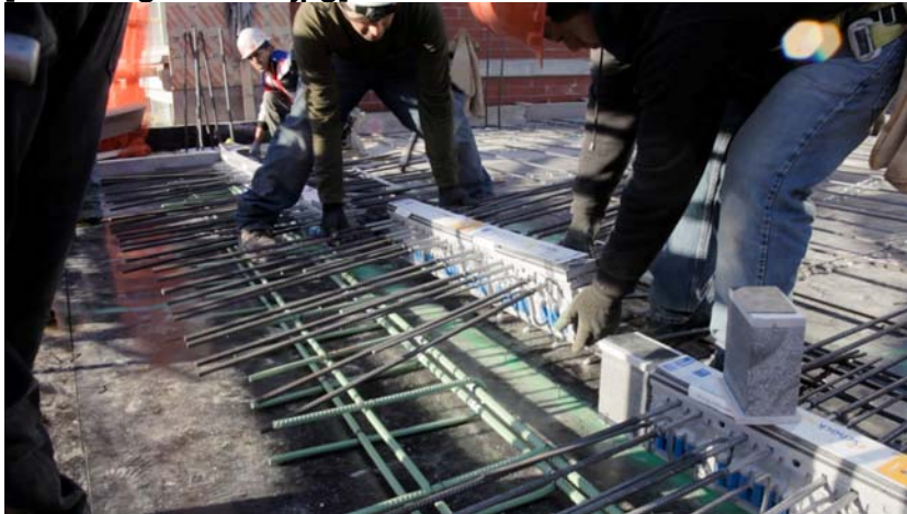
[Installing Isokorb.jpg]
