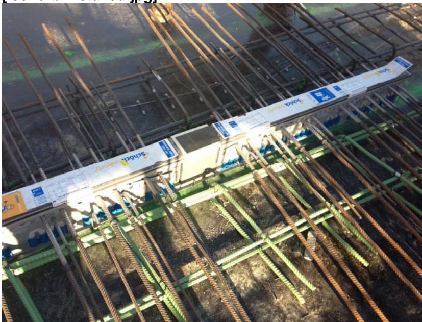
[Isokorb installed.jpg]
