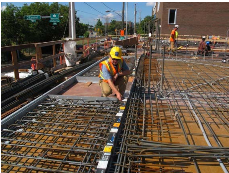
Simple, drop-in-place installation techniques for Schöck Isokorb ® , a load-bearing thermal break element for the thermal break of free cantilever balconies.
