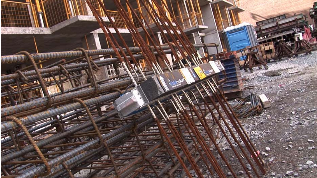
Schöck Canada's Isokorb thermal break element ready for installation.
