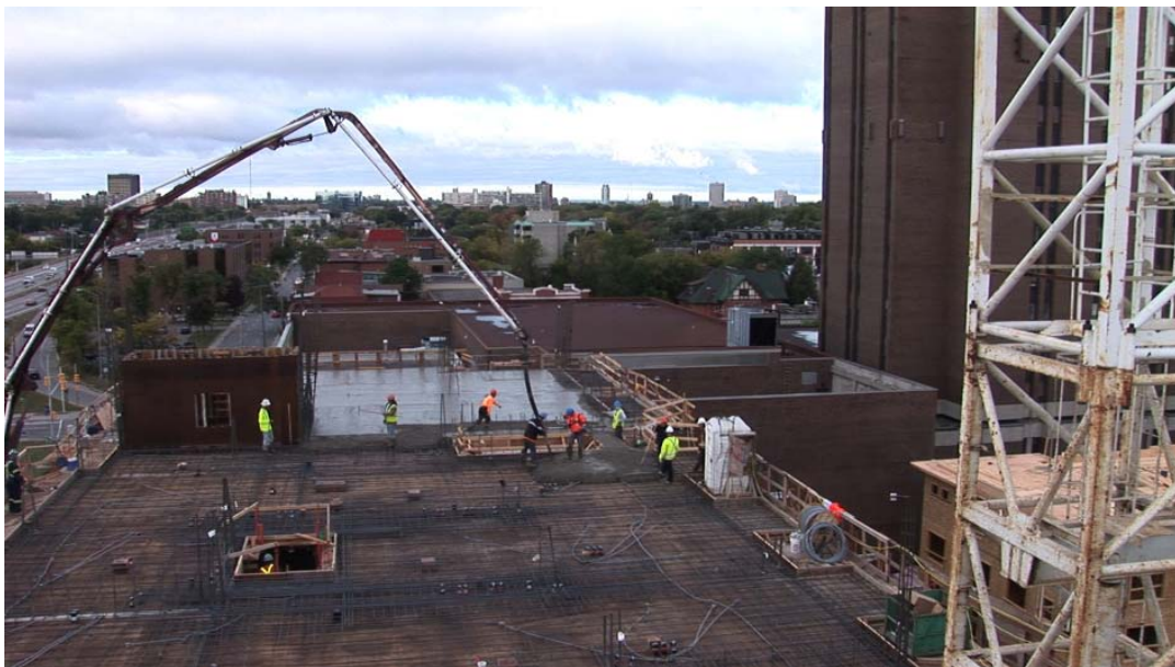
The Beaver Barracks redevelopment site located in downtown Ottawa.
